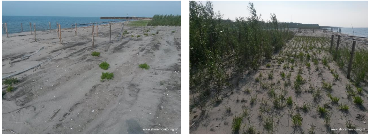
Figure 7. Left: section on foreshore pilot Houtribdijk with natural vegetation evolution. Right: planted section of the foreshore with four type of willows at the higher foreshore and reed. The photo also shows an enclosure in which the reed density is substantially higher due to the absence of grazing here.
